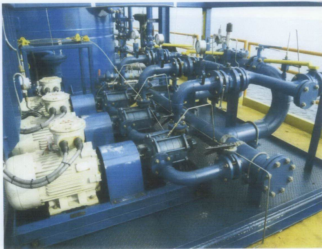
Figure 25: LPS High Pressure Pumps
