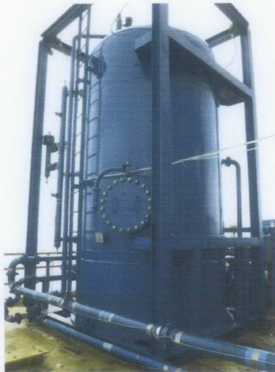
Figure 24: LPS Surge Tank
