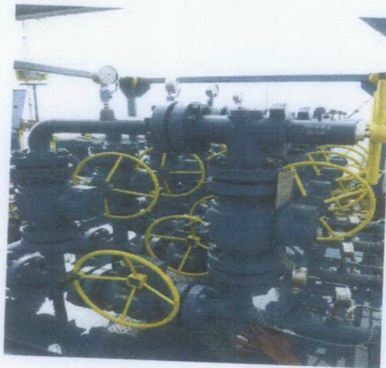
Figure 6: LPS Choke Manifold
