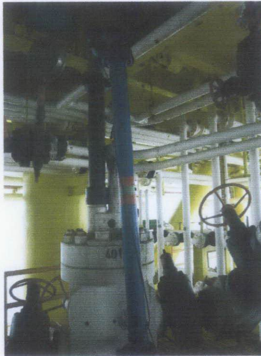
Figure 21: Wellhead Connection
