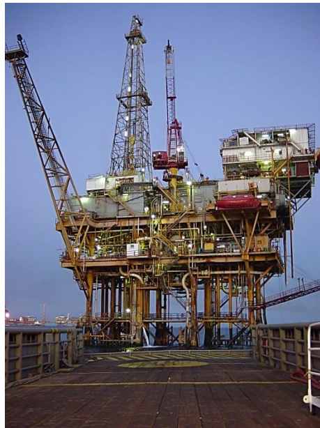
Figure 1.0.1: A fixed offshore platform.
