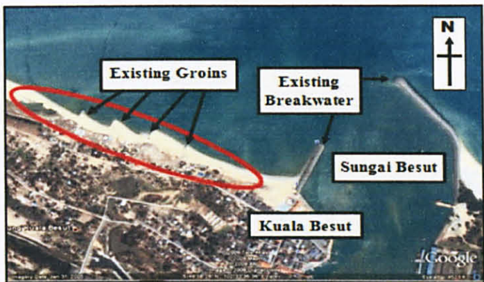
Figure 1.4: Rivermouth and the Existing Structures (2 Aug 2005)
