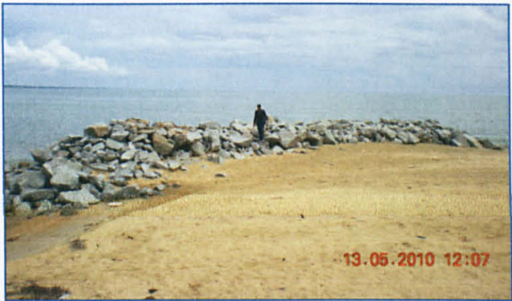
Figure 1.5: Location photo at groin of Kuala Besut
