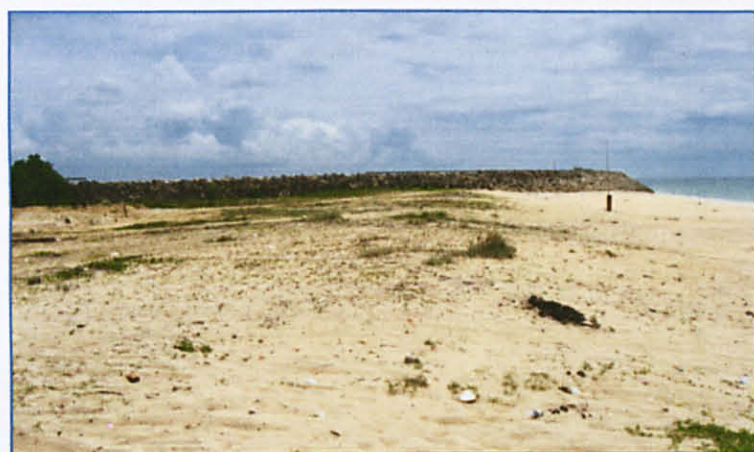
Figure 1.7: Location photo to the right of Kuala Besut right breakwater
