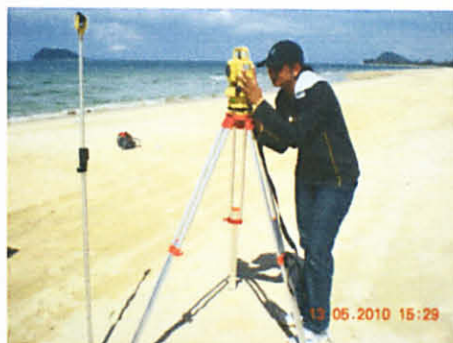
Figure 3.6: Slope measurement using the total station
