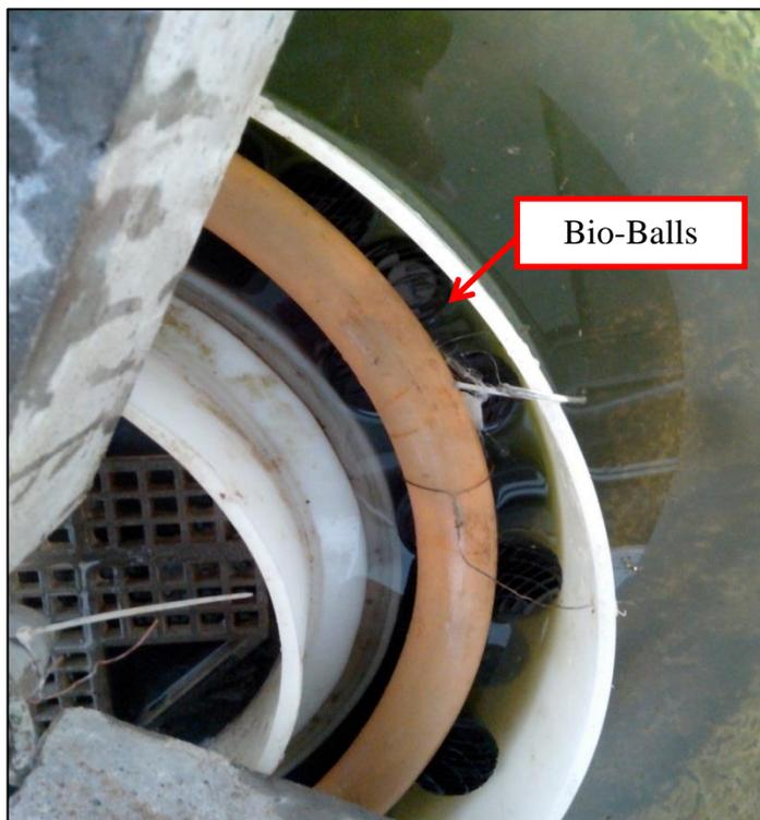
**Figure 15:** Installation of the Bio-Balls in the Anoxic Tank
