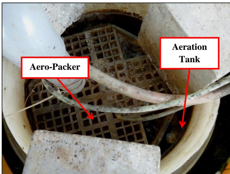
**Figure 13:** Top View of Aeration Tank after the Installation Aero-Packer
