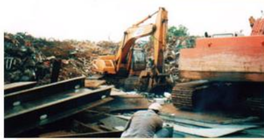
Welder at Work in Heng Hiap Metal.
