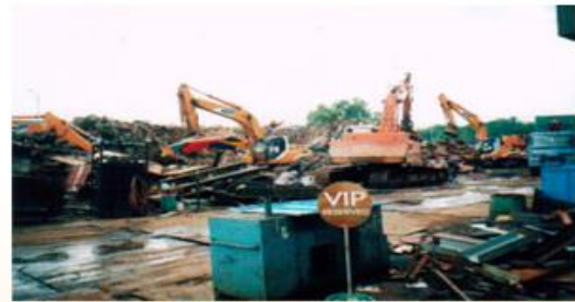
The Facilities and Machineries in Heng Hiap Metal.
