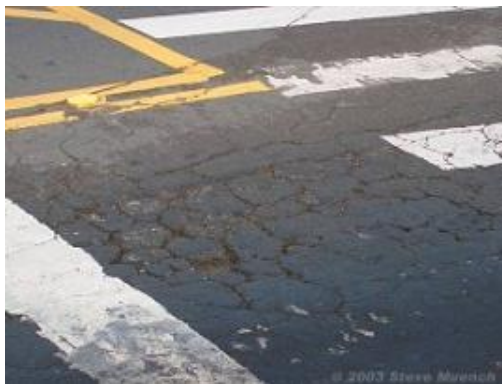
Figure 8 : Alligator Cracking
