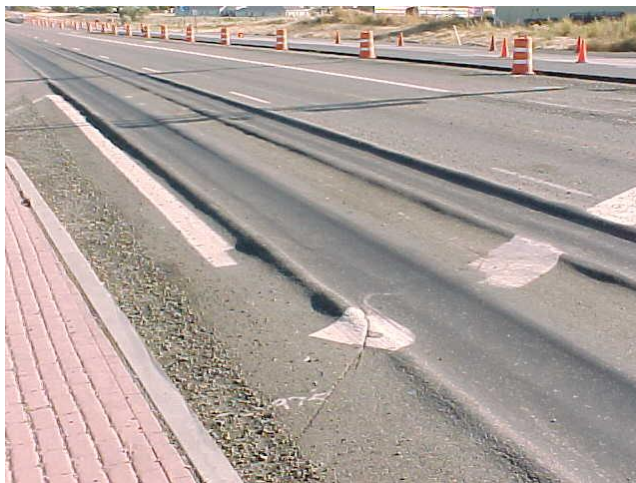
Figure 10 : Severe mix rutting
