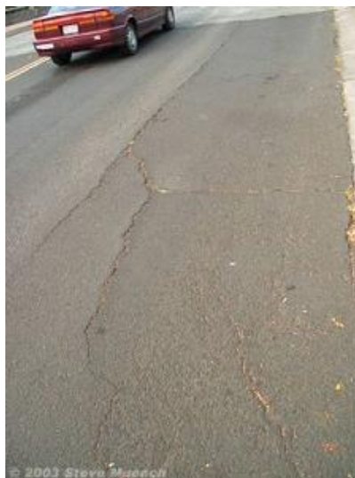
Figure 9 : Block Cracking
