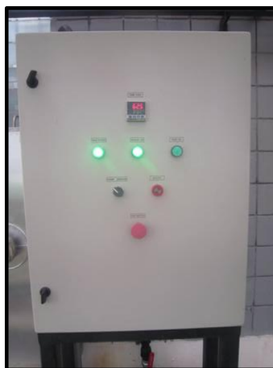
Figure 5 Hot Water System's Control Panel
