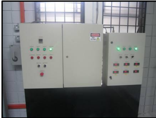
Figure 4 Gas Separation Unit's Control Panel
