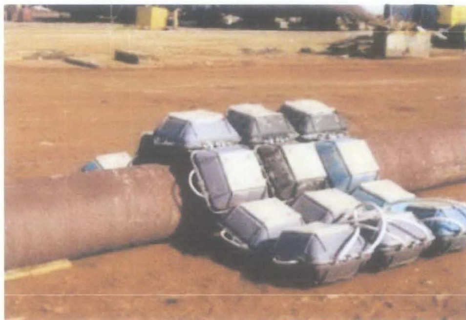
Figure 2: Secondary stabilization – concrete mattresses [13]
