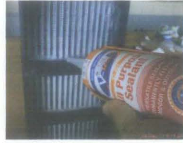
Figure 3.15: Sealing the joint with silicon sealant
