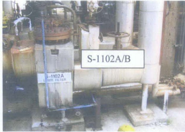
Figure 2.3: Basket Strainer S1102A/B (refer to Project Risk Assessment for HP Crude LSWR Rundown System Debottlenecking Project presented by Kamaruzzaman , 2008)
