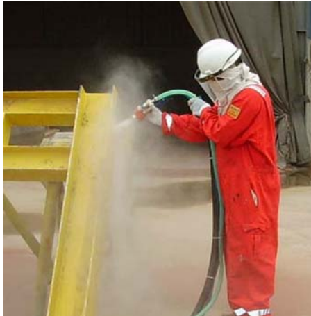
Figure 1.1: One of the coating procedures - blasting process on the offshore structure
