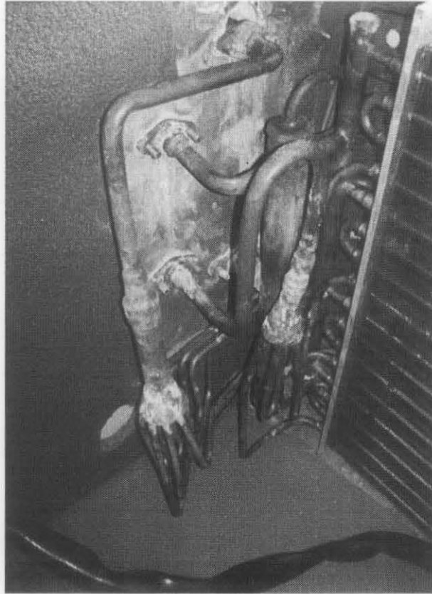
Figure 3.9: Distributor and header piping of the cooling coil and reheat coil
