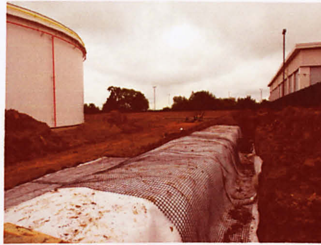
Earth bund lined with HDPE under surface
