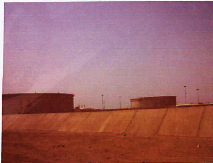
Earth bund lined with Concrete
