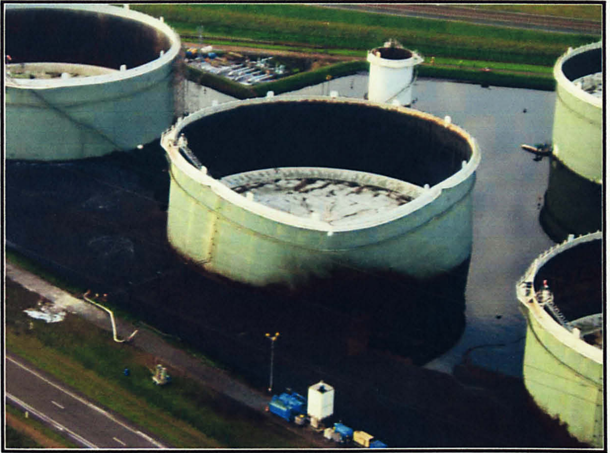
Figure (2.7): Picture of the situation in the bund the morning after the major accident
