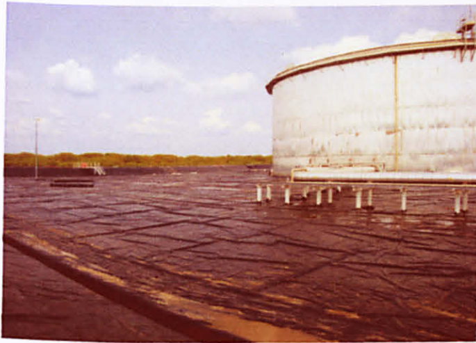
Earth bund lined with HDPE on surface
