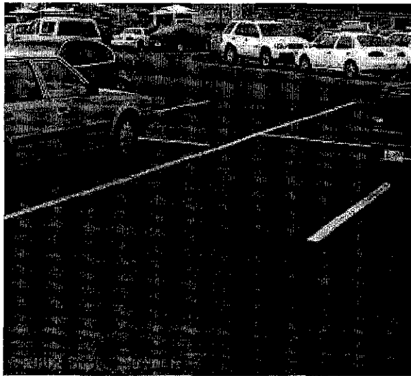
Figure 3: Fog Seal on the Right Hand Side
