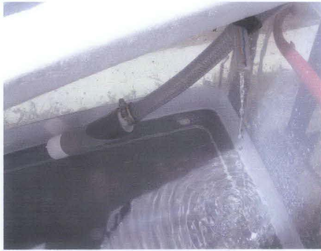
Figure 11: The pump (left side) and TES tank outlet (right side)
