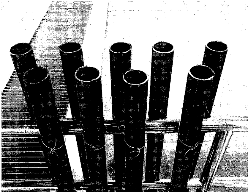
a) Bare steel tubes are tied and to be filled with grout.
