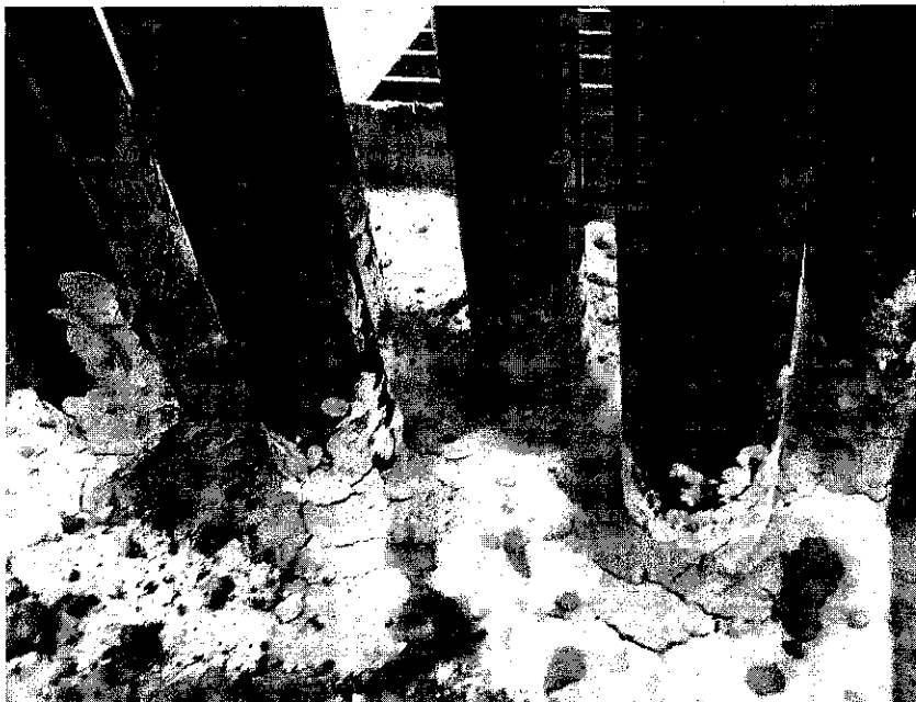
b) Bottom of the steel tubes are sealed with clay.
