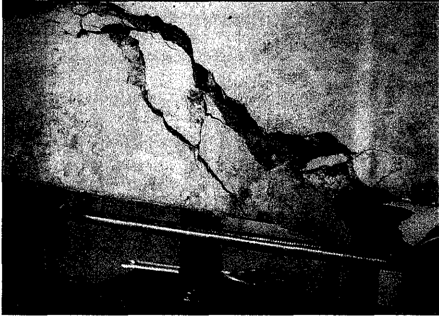
Fig 4-9: Crack Flow of Beam 2
