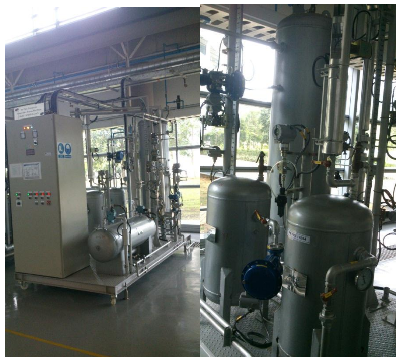
Figure 8 PID Pressure Control Pilot Plant
