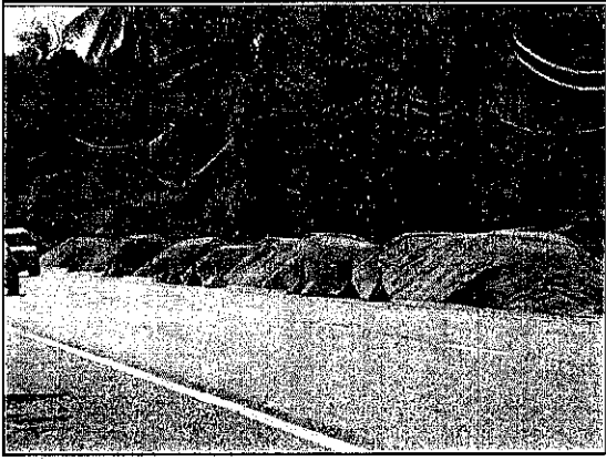
Figure 8.2d: Surcharge fills
