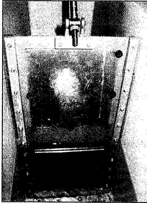
Figure 4.5: Movable overflow weir
