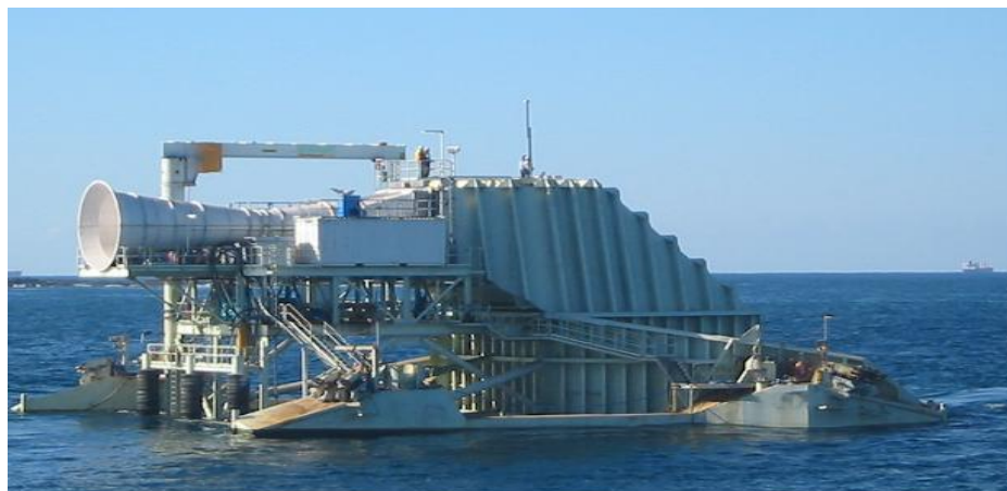
Figure 1.4: Oscillating water column (OWC) [2].
