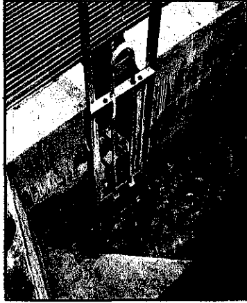
Figure 3. Manual screen bars (before rectified)
