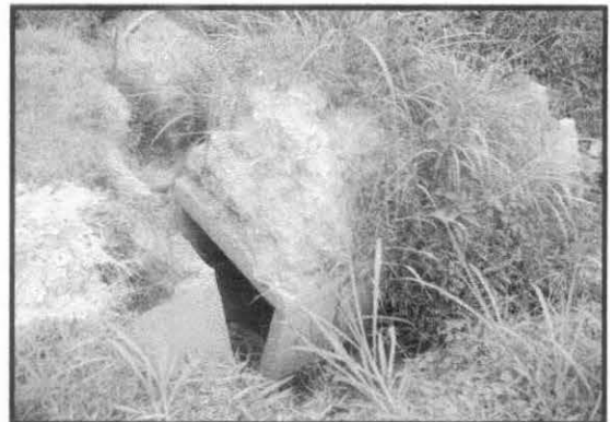
Figure 7 : Drain structure collapsed at site
