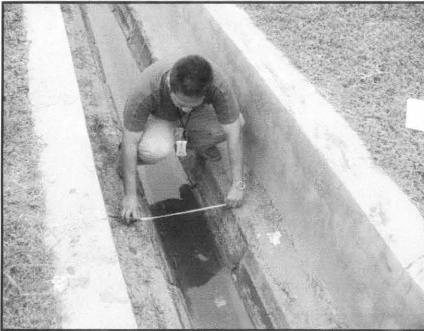
Figure 4 : Measuring the drain properties
