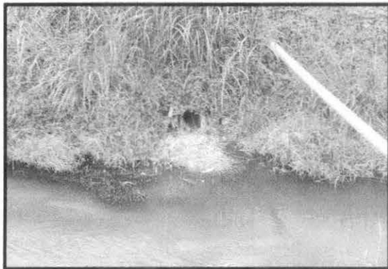
Figure 6 : Culvert covered by sediments and vegetation
