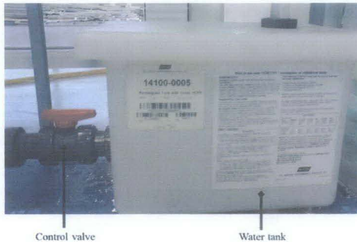
Figure 4.7 : Control valve & water tank of the system
