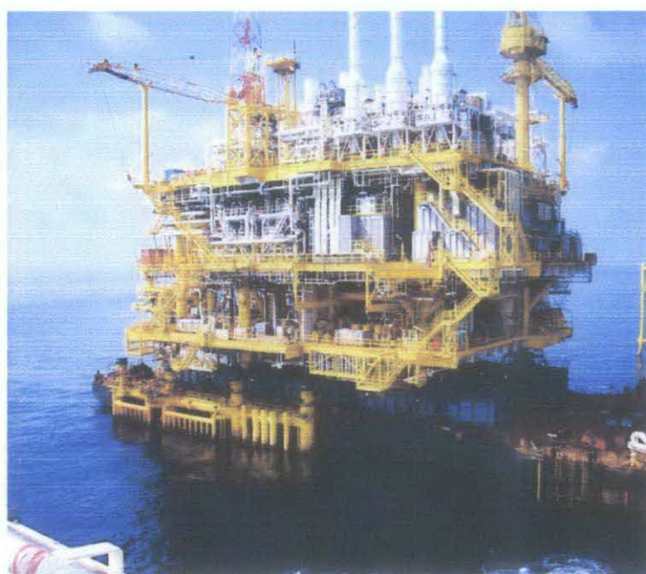
Figure 6: Arthit Deck – as the barge enters the jacket slot
