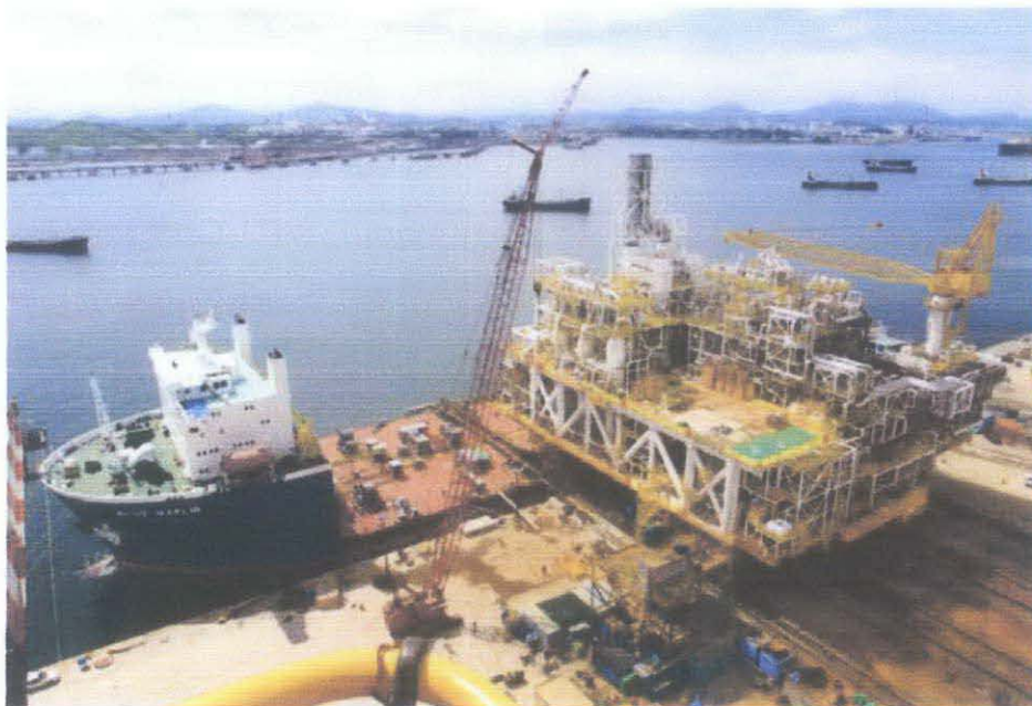
Figure 16: Skidded load-out
