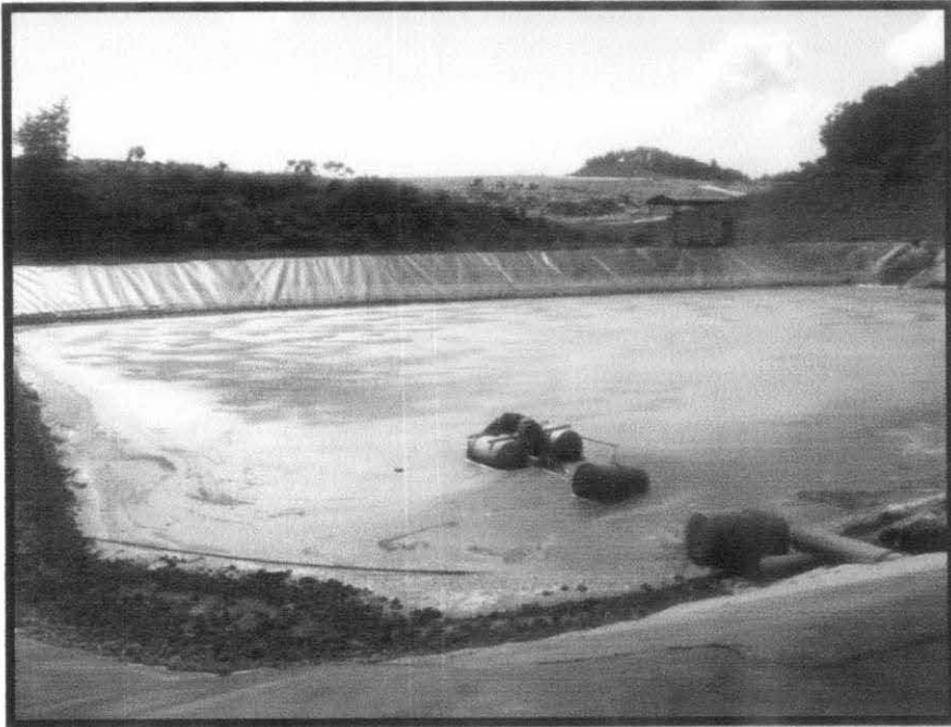
Figure 4 : Leachate pond at Bukit Tagar
