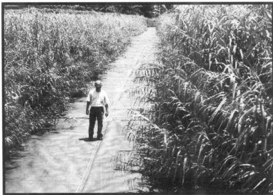
Figure 6 : Part of the extensive Reed Bed Polishing System
