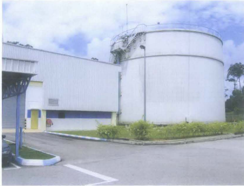
Figure 6: Thermal Energy Storage at District Cooling Plant
