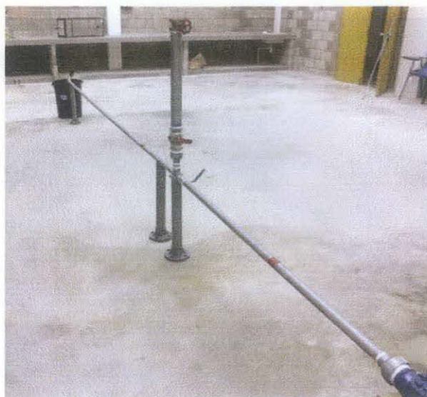
Figure 9: The galvanized steel pipe sections.
