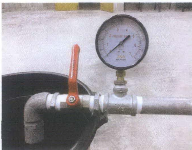
Figure 10: The pressure gauge.
