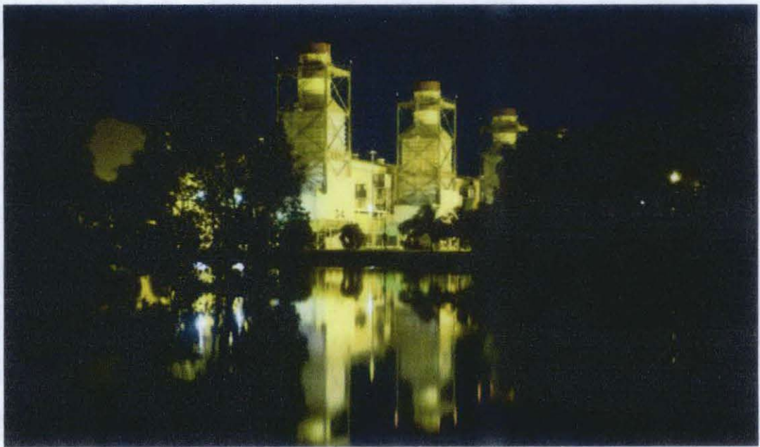
Figure 13: Port Dickson Power Plant [13]
