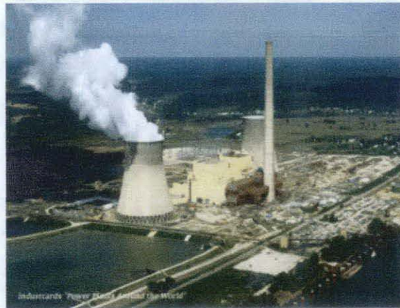
Figure 3: Coal Power Plant [8]
