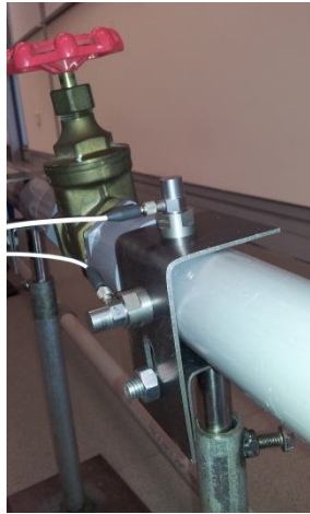
Figure 3.8: Accelerometer position on the pipe clamp support
