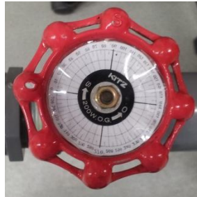
Figure 3.6: 360 degree scale on the valve handle
