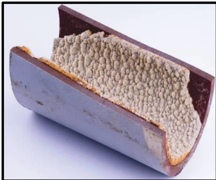
Figure 1: Hydrate layer in pipeline
