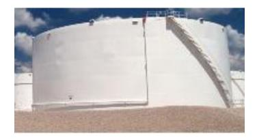
Figure 24: Floating Roof Tank.
