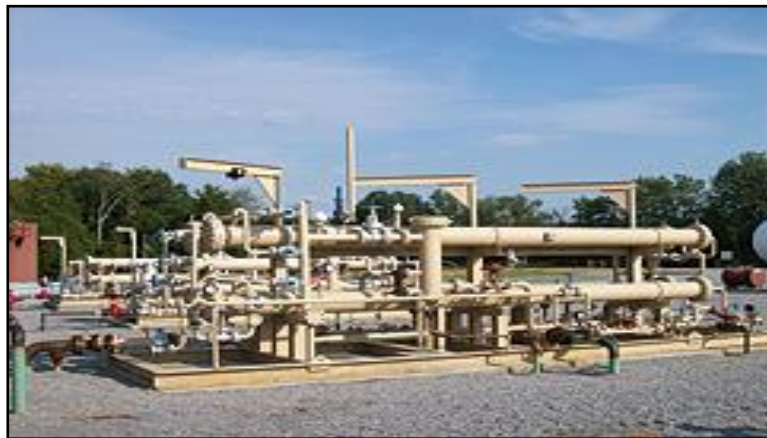
Figure 2. 2: NitroSep™ units upgrading high nitrogen gas in California
