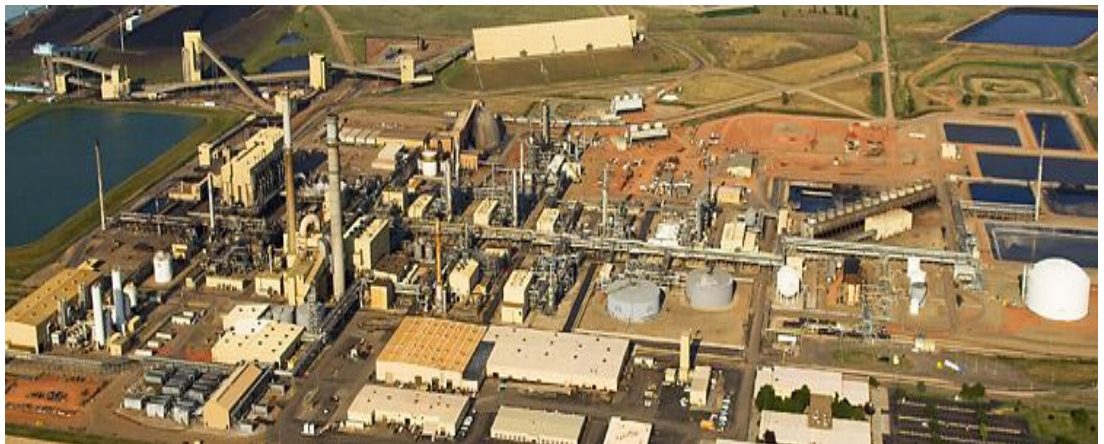
Figure 4.1: The Great Plains Synfuels Plant
