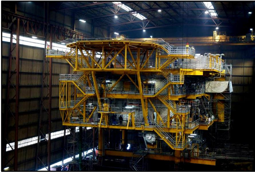
Figure 2.1: Topside Hasdrubal 'A' by Heerema Fabrication Group (HFG). Adapted from Rigzone.com
