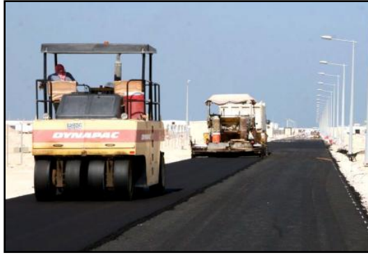
Figure 2.7.1: Sulfur-modified asphalt application during the mix lay down process (Ras Laftan Industrial City (RLIC), Qatar in October 2007) [ 3 ]
