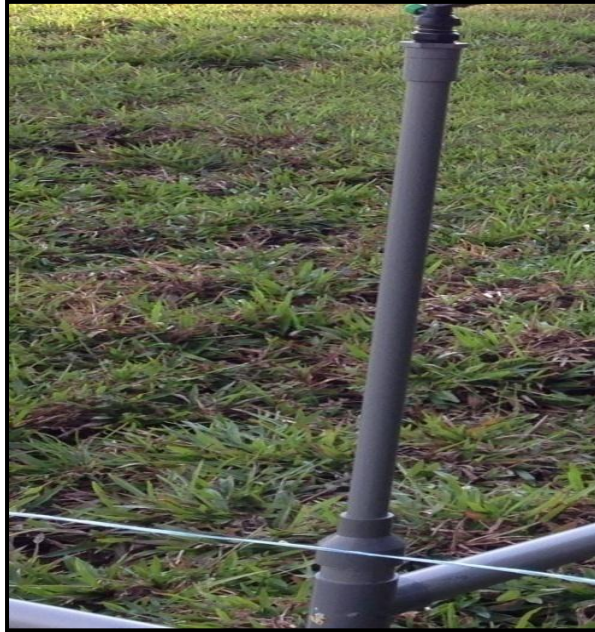
Figure 3.5: PVC Pipes 20 mm Diameter for Sprinkler Riser
