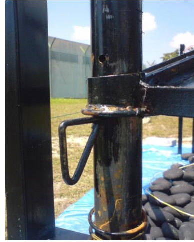
Figure 6.6: Metal hook for canopy adjust
