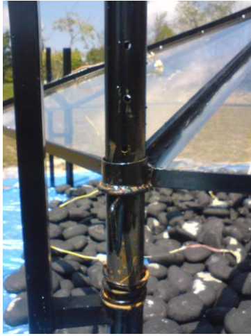
Figure 6.5: Canopy leg support with pre-drilled holes
