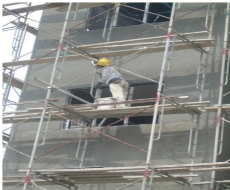
Figure 9: Worker did not wearing PPE and no tag is put at scaffolding
