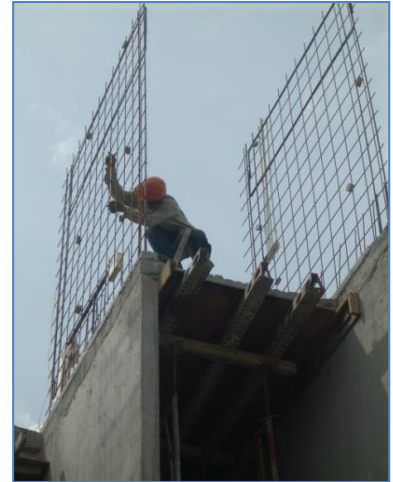
Figure 10: The worker didn't wear full body harness when doing the construction activity at height more than 6 feet
