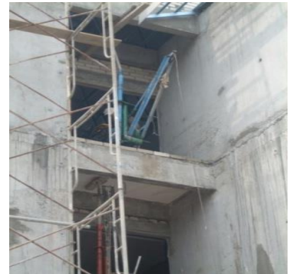
Figure 10: The worker didn't wear full body harness when doing the construction activity at height more than 6 feet
