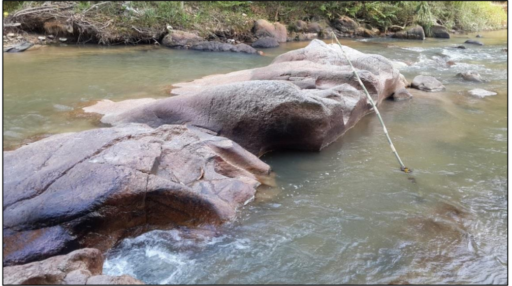
Figure 21: More fractures in the granite that has been widened by flowing water
