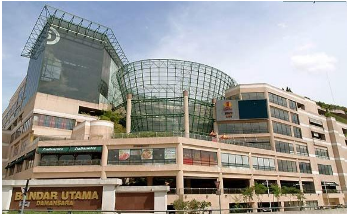
Figure 39: 1 Utama Shopping Mall in Kuala Lumpur
