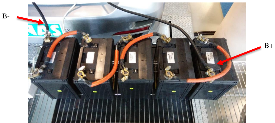
FIGURE 14: Series-Connected 12V Lead Acid Batteries
