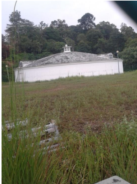
Figure 6: UTP Water Storage Facility
