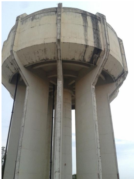
Figure 7: UTP Water Tank Tower
