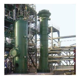
Figure 2.3-2 Installed Hydrate SeparatorTM for JT-LTX system (TwisterBV, 2011).
