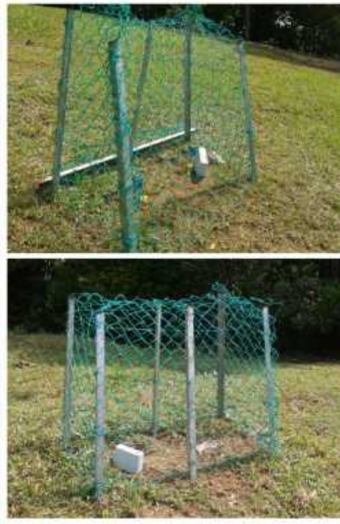
Figure 3.3: The tensiometers installed at the site
