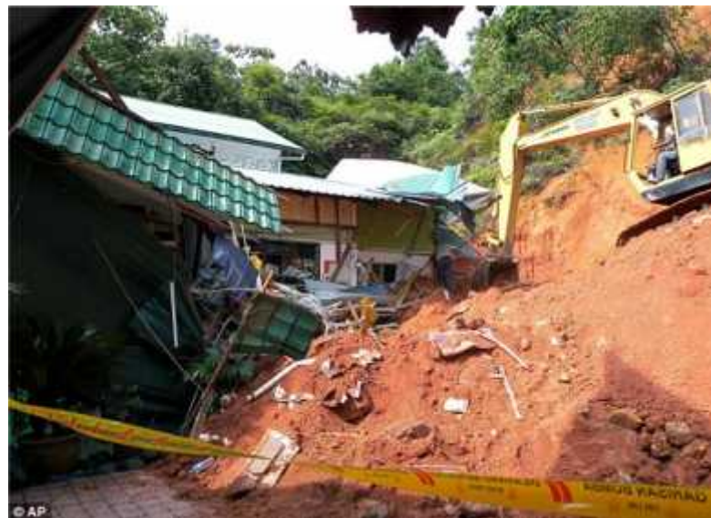
Figure 1.1: Massive landslide occurred in 2011 in Hulu Langat due to heavy rainfall
