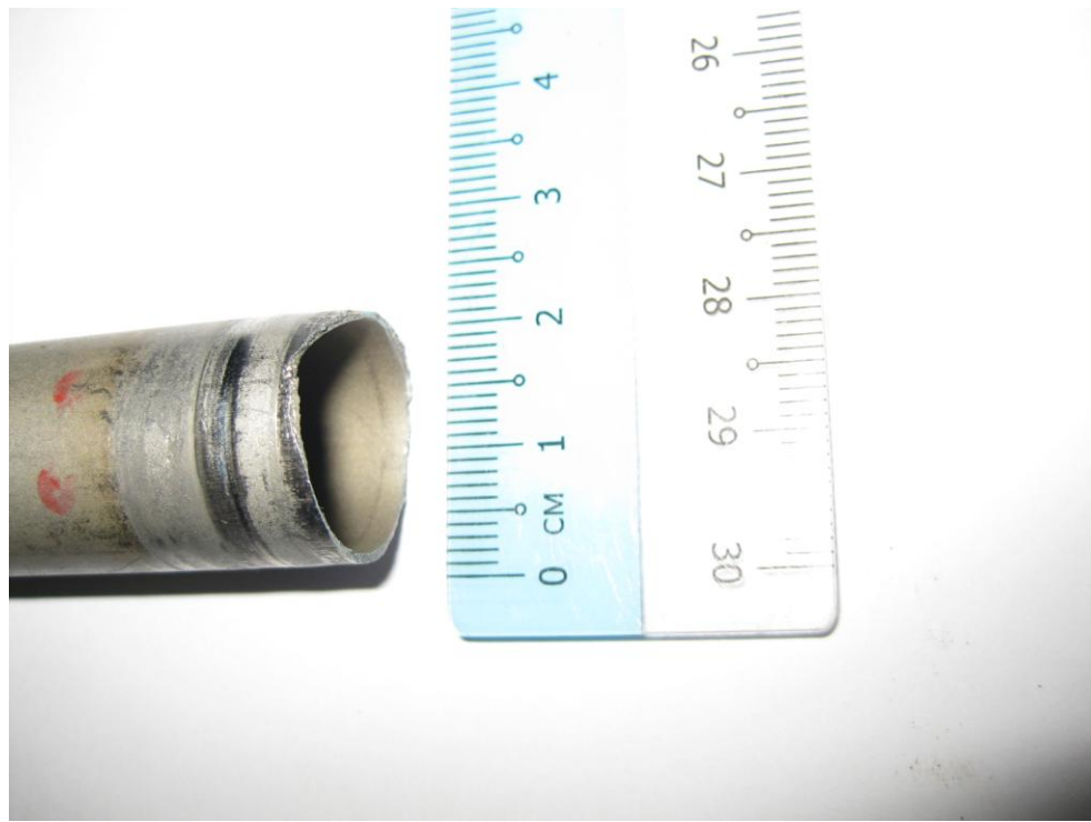
Appendix 4: Broken side of the stainless steel tubing.
