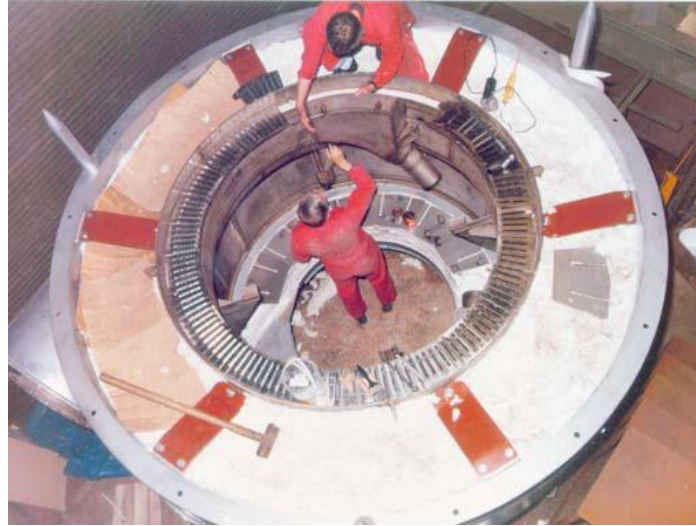
Figure 1.4: TORBED, a commercial version of swirling bed, being assembled on site [7].
