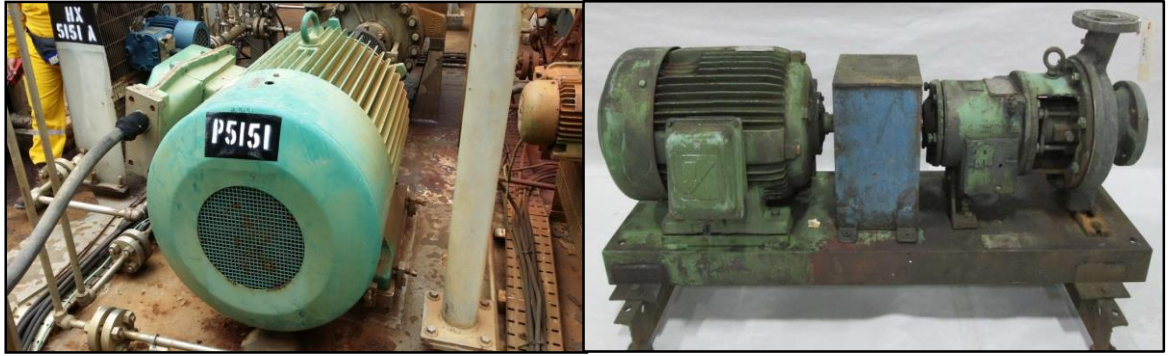
Figure 1: Condensate Transfer Pump: Centrifugal Type
