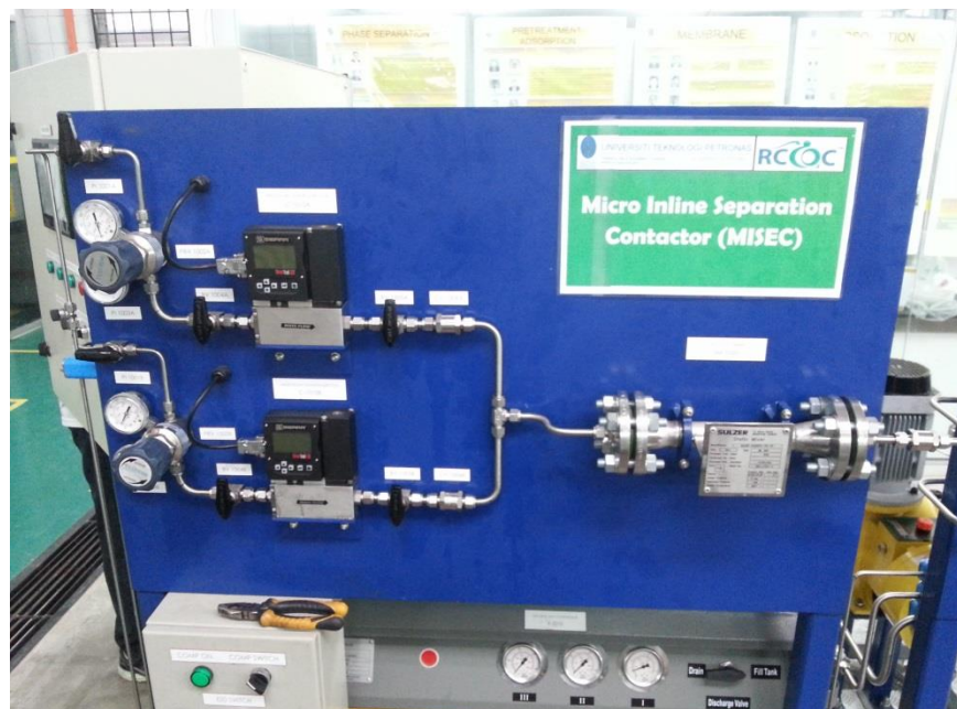
Figure 29: Flow Controller for gas feed
