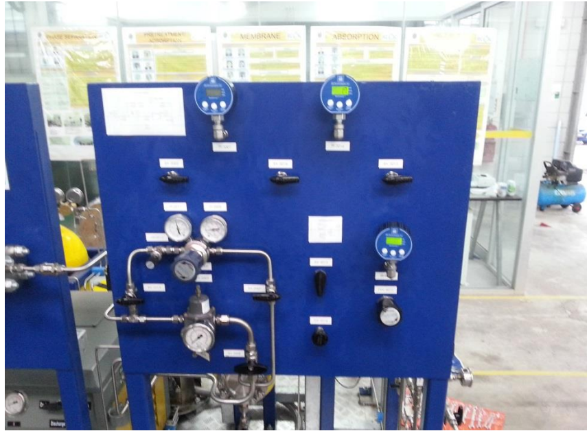
Figure 30: Pressure relive valve and Ball valve controller
