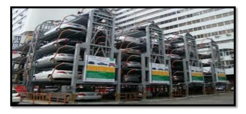
Figure 2.6: Rotary Parking System
